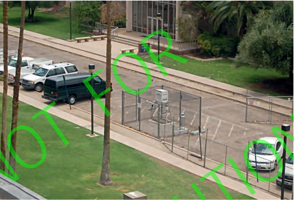
Figure 3.1: U.S. Historical Climatology Network weather station used to collect climate data. This station is located in a parking lot at the University of Arizona in Tucson. The station was previously located in a grassy area, but researchers moved the station as the campus grew. Photo by Anthony Watts.
